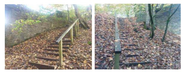
The twin steps are followed by fairly steep surfaced incline leading to the valley floor. The surface is made from crushed limestone which is firm underfoot but covered in leaf litter in the autumn. The gradient is 15% from the valley floor.
