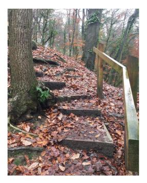
The bridge leads to approximately 52 steps with timber risers and deep steps of crushed lime stone with partial handrails. This gradient is steep and long at over 20%.
